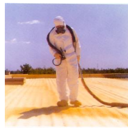
Spray heat insulation
